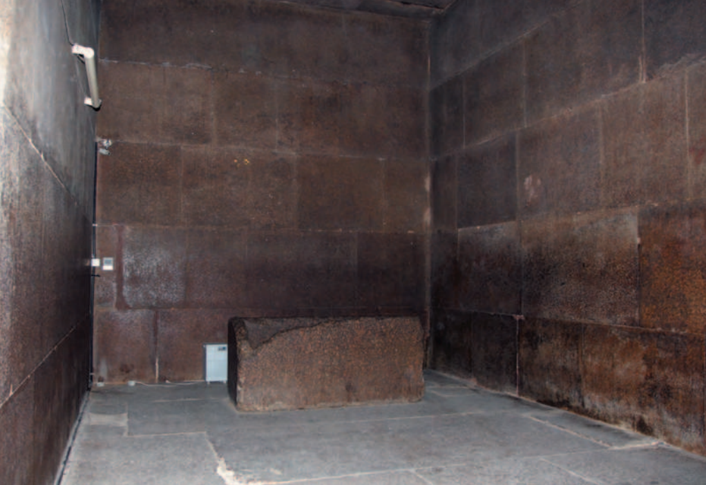
Burial chamber of Khufu in Giza: this room is built entirely of red granite from Aswan, as is the sarcophagus chest (the lid is missing).
